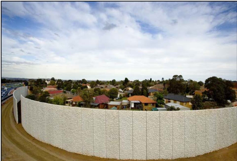
Noise Walls: Cantilever
