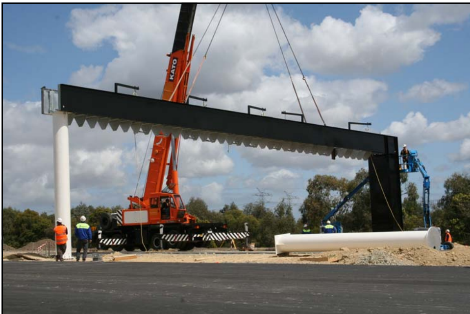
TP4 – Erection of first tolling gantry
