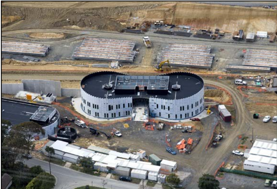
Progress on ELOC building
