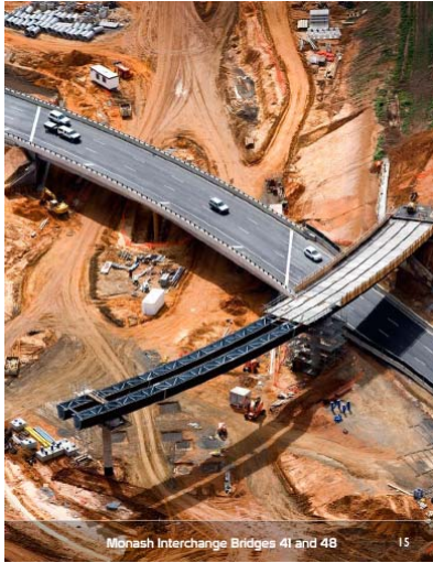
Monash Interchange Bridges 4I and 4B 15
