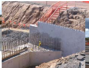
Abutment beam poured
