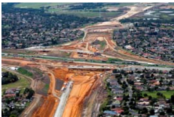
Aerial view of interchange Under construction
