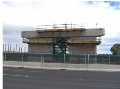
Pier construction with falsework
