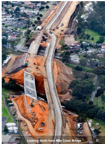
Looking North from Mile Creek Bridge 25
