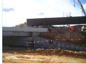
EastLink S/B Entry Ramp over EastLink 1800mm Super-Ts Continuous pier diaphragm
