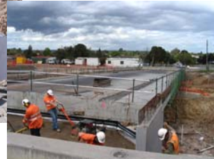
Insitu concrete fenderwall poured connecting to wingwall
