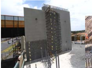
Wingwall Lifted into place
