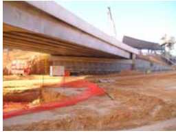
EastLink S/B Entry Ramp over EastLink 1800mm Super-Ts Continuous pier diaphragm
