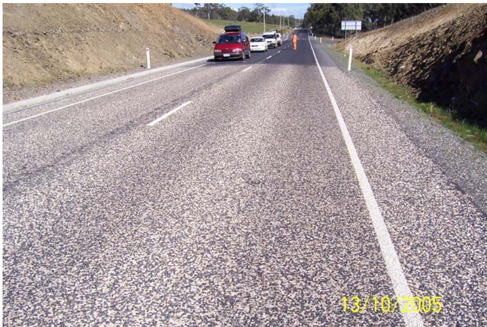
Figure 7. General view of the 50/50 blend and Control (Basalt) at the back.
